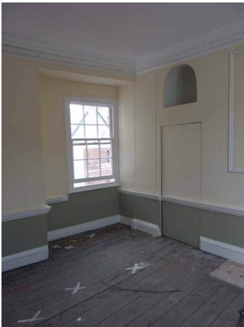
Refurb under way
